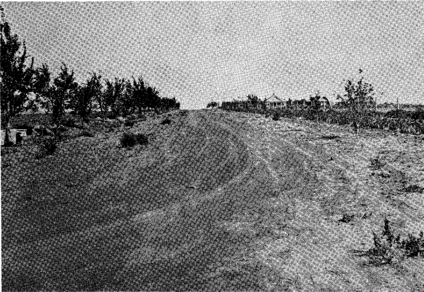
Fig. 11.-Main drive on station as seen in 1918.
