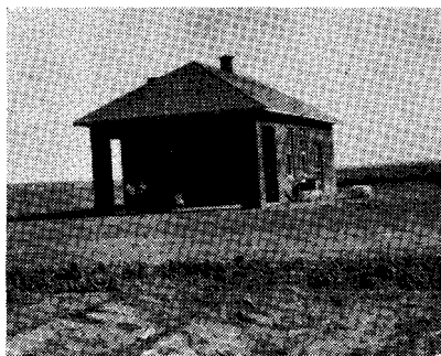
Fig. 4.-Office Building (1913). Used until 1948.
