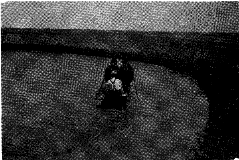
Fig. 30.-Puddling Reservoir-1914. This was necessary to reduce losses by seepage. Even with frequent puddling, 6 to 10 inches of water were lost each day.
