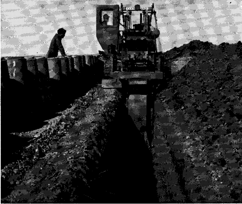
Fig. 31.-Concrete pipelines were installed for irrigation on the main station in 1954 and 1955. These lines consist of 1,681 feet of 15 inch line and 2,797 feet of 18 inch line. A total of 2,682 feet of 15 inch line was constructed at the irrigation project north and west from Holcomb in the fall of 1956. The value of underground distribution was recognized as early as 1914 when a request was made for such a system.
